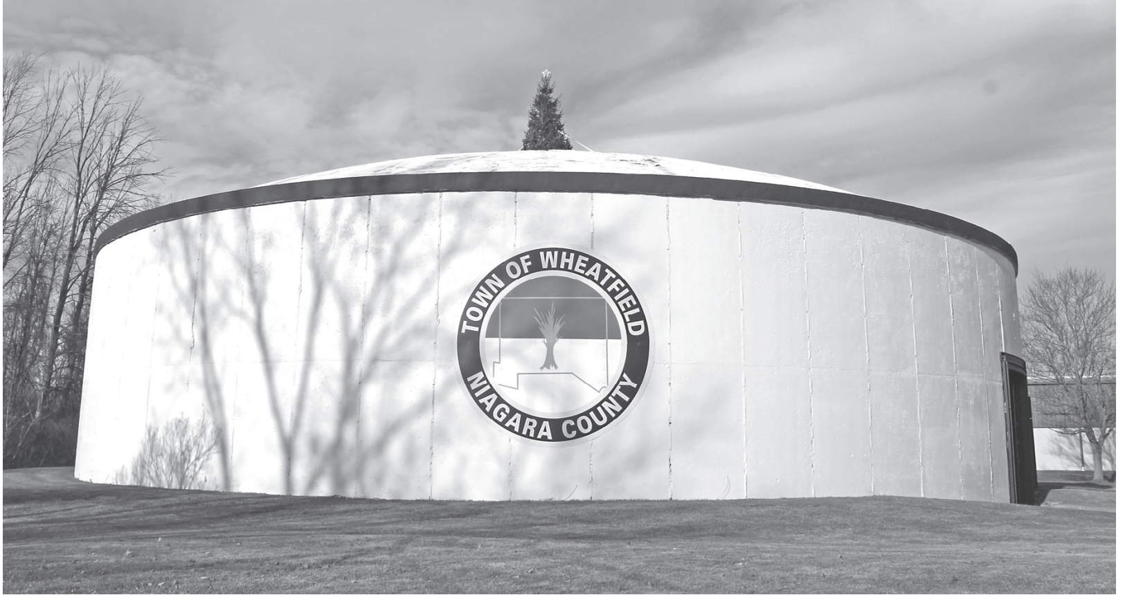
The water tank sports a huge new logo at the Water & Sewer Department at 3113 Niagara Falls Blvd., Wheatfield. (Photo by Karen Carr Keefe)
